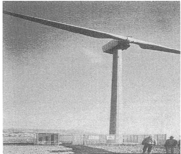
Fig. 2 3MW wind machine in Orkney, Scotland
