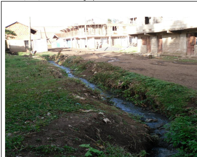
Figure 3: Domestic wastewater flowing in open ditches which finally discharge into Kiu River
