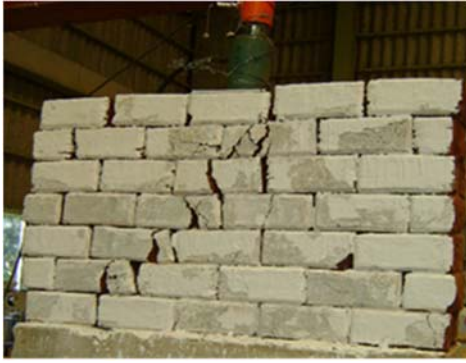
Figure 9: (a) Failure of 2% MSWA
